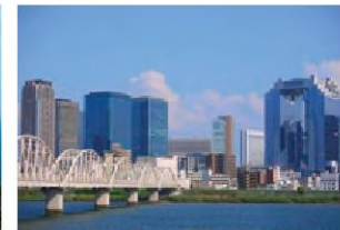
Distant view of Umeda (Osaka)
