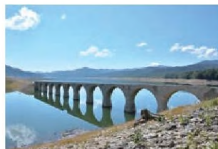
The Concrete Arch Bridge of the Shihoro Line
