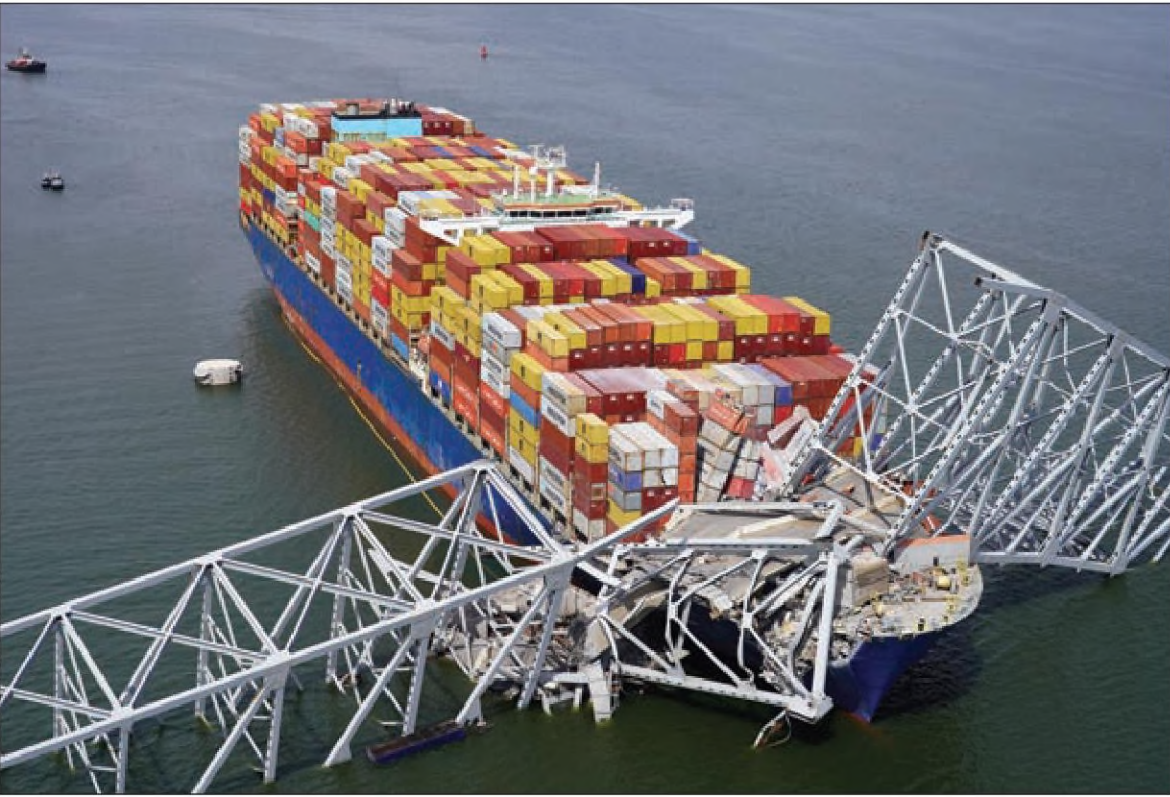
An aerial view of the Dali cargo vessel, which crashed into the Francis Scott Key Bridge, causing it to collapse, in Baltimore, Maryland, on Tuesday. At least six people were unaccounted for and presumed dead. REUTERS See story, page 7
