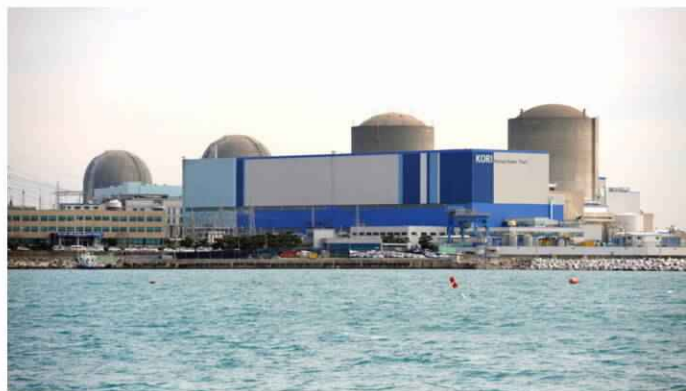
The Kori Nuclear Power Plant, Busan, South Korea, February 2008 | Source: Wikimedia Commons
