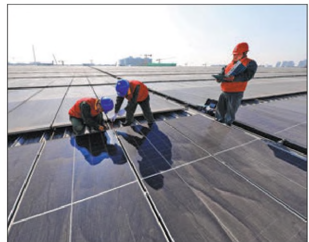
Technicians conduct safety checks on rooftop photovoltaic panels in Yiwu, Zhejiang province, in December. SHI BUFA / FOR CHINA DAILY
