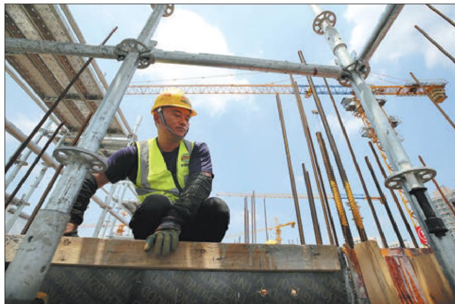
An employee of China Railway 24th Bureau Group Corp works at the Pengyi Community redevelopment project in Shanghai in May. FANG ZHE / XINHUA
