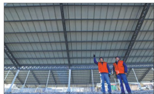
Workers check the PV panels installed at a stock farm in Zhangye, Gansu province, on Jan 4. PROVIDED TO CHINA DAILY
