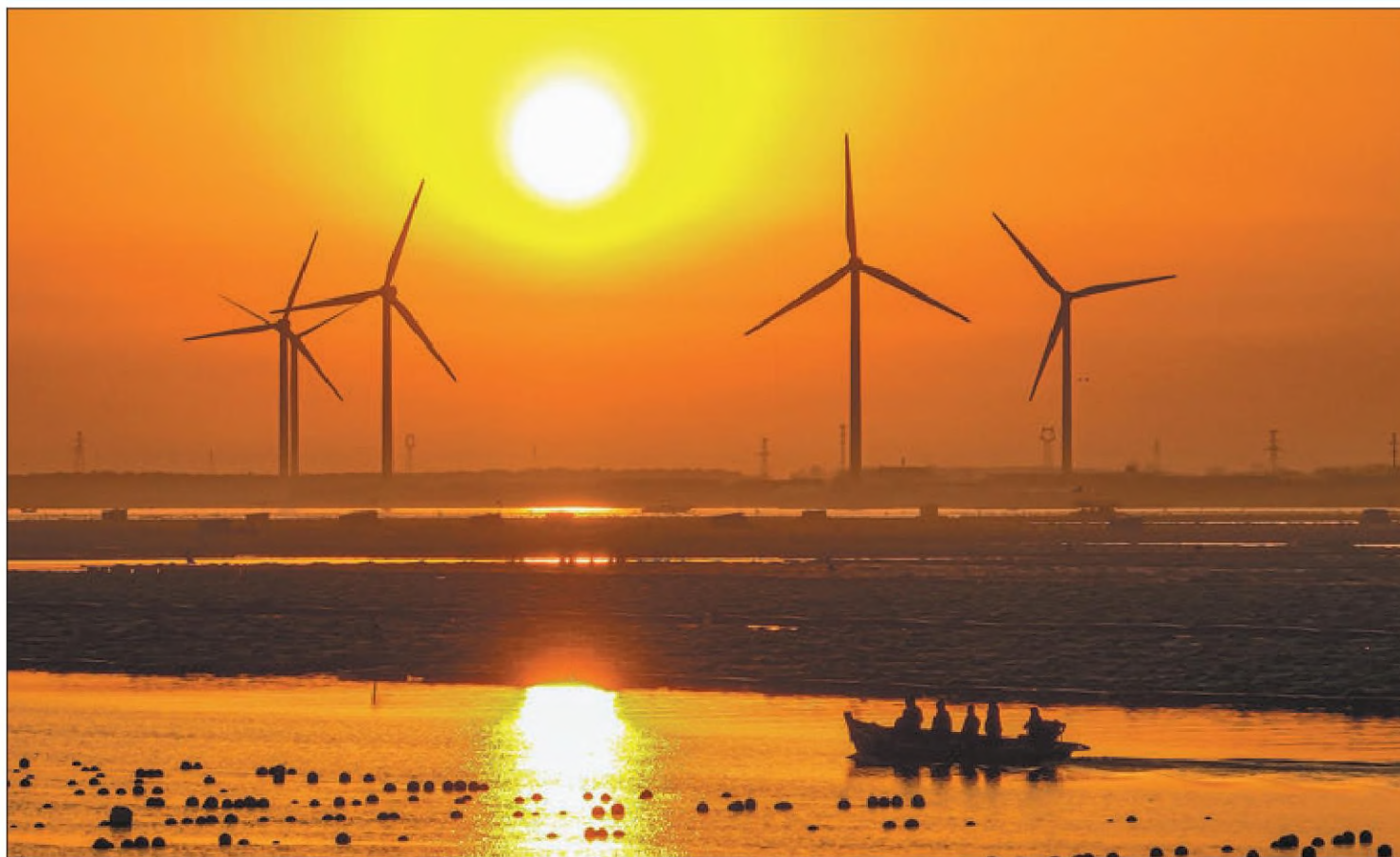
Wind turbines in the distance are at work before sunset in Rongcheng, Shandong province, on Jan 6. LI XINJUN / FOR CHINA DAILY
