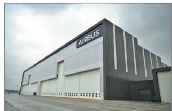
European aircraft manufacturer Airbus' life cycle services center is put into operation in Chengdu, Sichuan province, on Jan 24. LIU KUN / XINHUA
