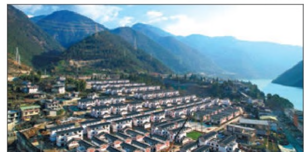
An aerial photo shows a newly built village for earthquake-affected families in Beitou village in Luding county, Sichuan province, on Jan 25. YANG JIN / XINHUA
