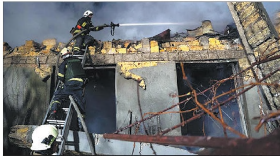
Firefighters work on the site of a burning building destroyed during an attack in Odesa on Friday. UKRAINIAN EMERGENCY SERVICE VIA ASSOCIATED PRESS
