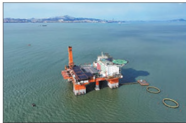
A view of an offshore solar platform off Yantai, Shandong province, in November. TANG KE / FOR CHINA DAILY
