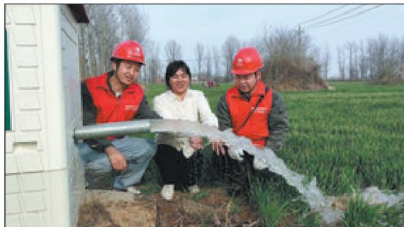
Employees of State Grid Queshan Power Supply Co check a facility in Queshan county, Henan province. ZHANG YONGSHENG / FOR CHINA DAILY
