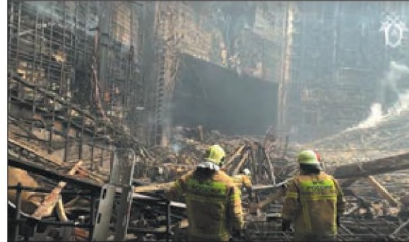
Firefighters work inside the gutted Crocus City Hall concert venue in suburban Moscow, Russia, on Saturday. Search operations continued inside the damaged building. INVESTIGATIVE COMMITTEE OF RUSSIA VIA AP
