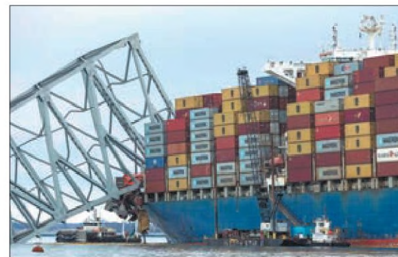
Wreckage from the collapsed Francis Scott Key Bridge rests on the cargo ship Dali on Monday, as efforts begin to clear the debris and reopen the Port of Baltimore. TASOS KATOPODIS VIA AGENCE FRANCE PRESSE
