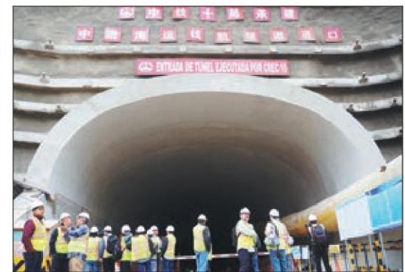
The tunnel gate to Chancay port facilities, is still under construction, on the Peruvian coast, on Aug 22. The port is being built by COSCO Shipping from China. CARLOS GARCIA GRANTHON / GETTY IMAGES
