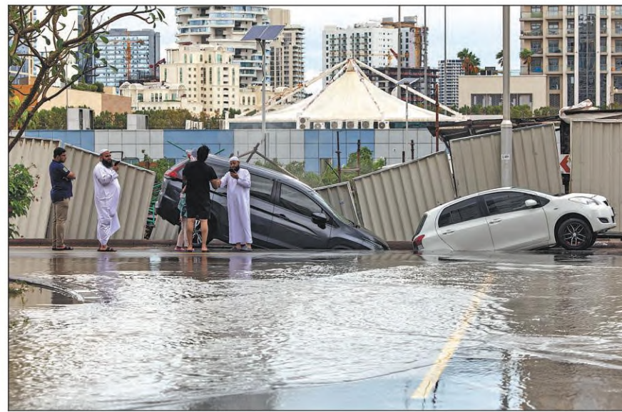
A portion of a road collapses in Dubai, the United Arab Emirates, after heavy rainfall on Tuesday, damaging vehicles. Authorities and communities across the UAE were clearing debris on Wednesday after at least one person died in a rare torrential storm. CHRISTOPHER PIKE VIA GETTY IMAGES
