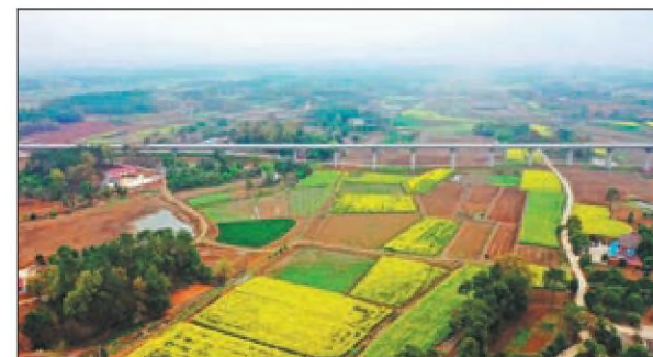
An aerial view of the Wuhan-Yichang section of the Shanghai-Chongqing-Chengdu High-speed Railway. China Railway 24th Bureau Group Corp, a State builder participating in the construction of the HSR, said girder installation of the Yichang section in Hubei province was completed last week, a milestone for the key HSR project that is being built along the Yangtze River. PROVIDED TO CHINA DAILY
