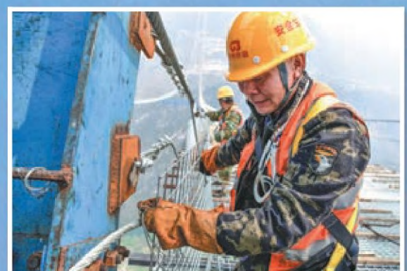
Workers on the bridge tower.
