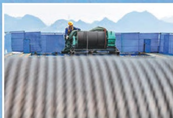
A worker on the bridge tower.
