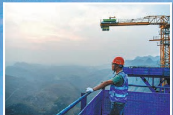
An engineer checks the progress of the bridge on March 26.
