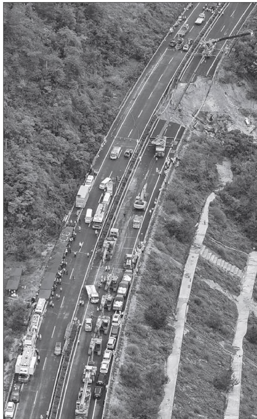
An aerial view of the collapsed section of highway in Meizhou, Guangdong province, that killed 24 people and injured 30 others when it gave way on Wednesday morning. The survivors, none with life-threatening conditions, are receiving treatment in hospitals. XINHUA
