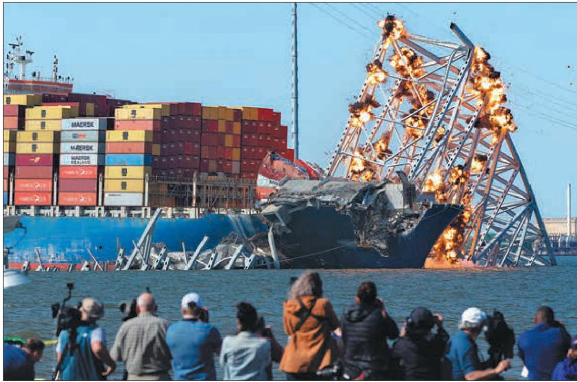
Explosives are detonated on Monday to bring down the Francis Scott Key Bridge, which partially collapsed after being hit by the container ship Dali on March 26, in Baltimore, the United States. The bridge was demolished to free the vessel that had been trapped under it for seven weeks. MARK SCHIEFELBEIN / AP
