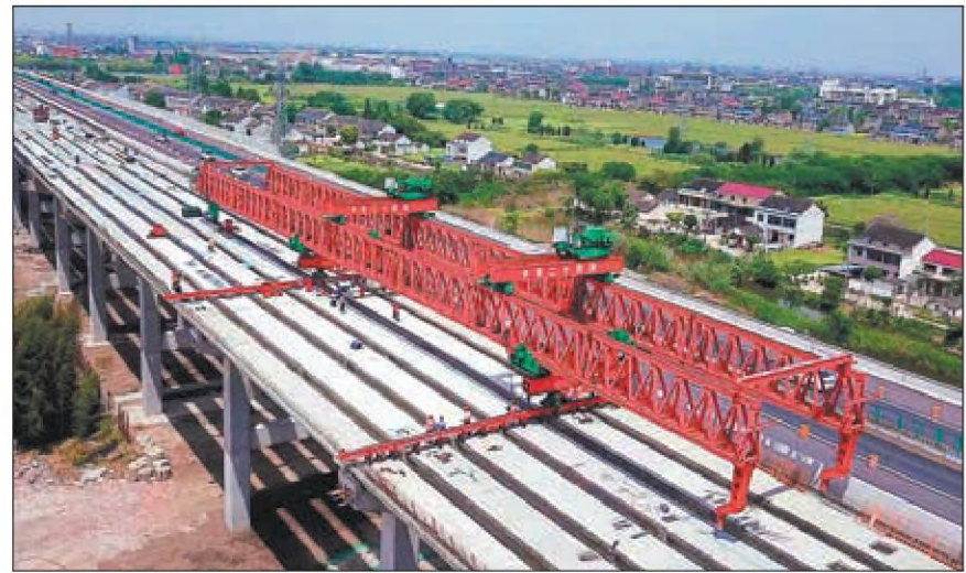
A drone image shows the construction site of a highway expansion project in Jingjiang, Jiangsu province, last week. Builders with China Railway 24th Bureau Group Corp completed installation of box girders of a major bridge, a milestone in the expansion project of the Pingchao-Guangling section of the Shanghai-Xi'an Expressway, which aims to enhance coastal-inland links. PROVIDED TO CHINA DAILY
