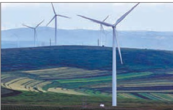
Rows of wind turbines stand on the Huitengxile Grassland in Chahar Youyi Zhongqi, Ulanqab, Inner Mongolia autonomous region, in August. TANG DEHONG / FOR CHINA DAILY
