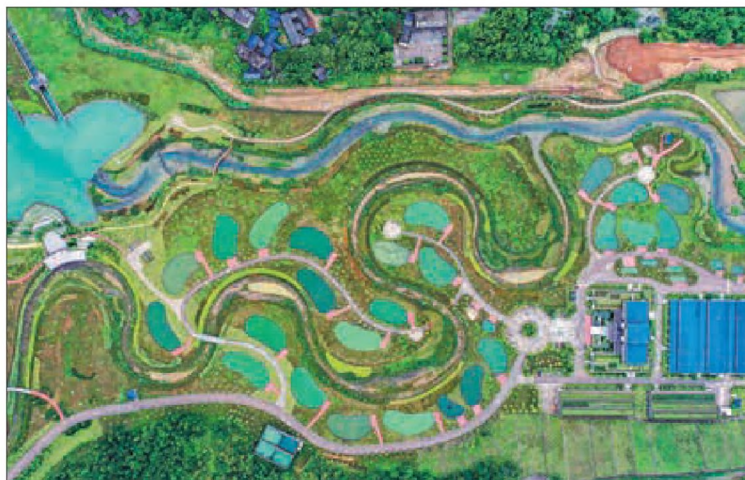
An overhead view of the fish ladder along the Nanmu auxiliary dam of the Datengxia Gorge Water Conservancy Hydropower Project in Guiping, Guangxi Zhuang autonomous region. It is one of two fish ladders built along with the project. CAO YIMING / XINHUA
