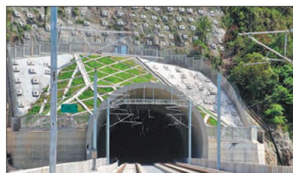
A tunnel on the Hangzhou-Wenzhou High-speed Railway in Zhejiang province. Built by China Railway 24th Bureau Group Corp, the HSR has started joint testing, marking countdown to its full operation. PROVIDED TO CHINA DAILY
