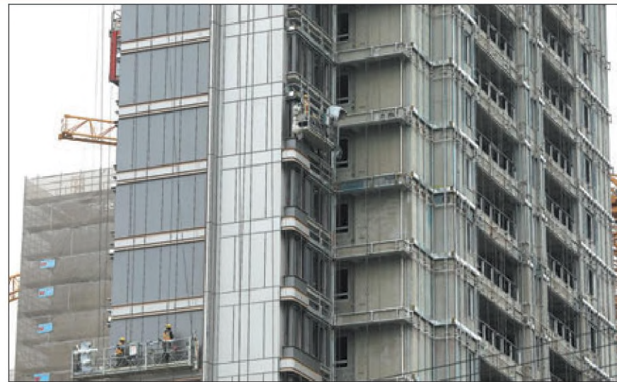
A property construction site in Shanghai. PROVIDED TO CHINA DAILY
