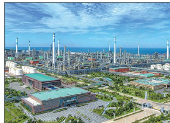
An aerial view of Hengli's industrial park in Dalian, Liaoning province. PROVIDED TO CHINA DAILY
