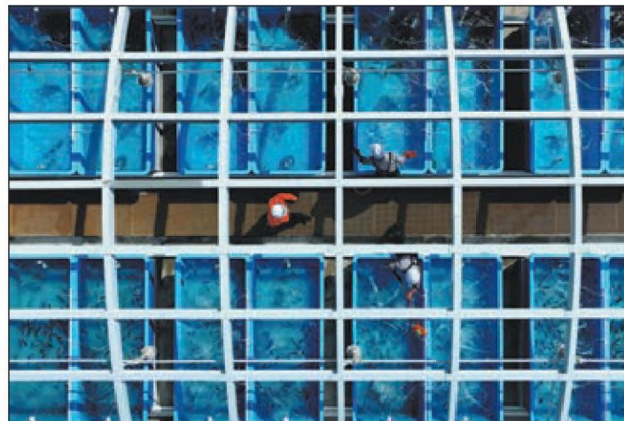
An aerial view of the Guangdong Dapeng LNG terminal in Shenzhen, Guangdong province, in January. WANG XIAOKE / FOR CHINA DAILY
