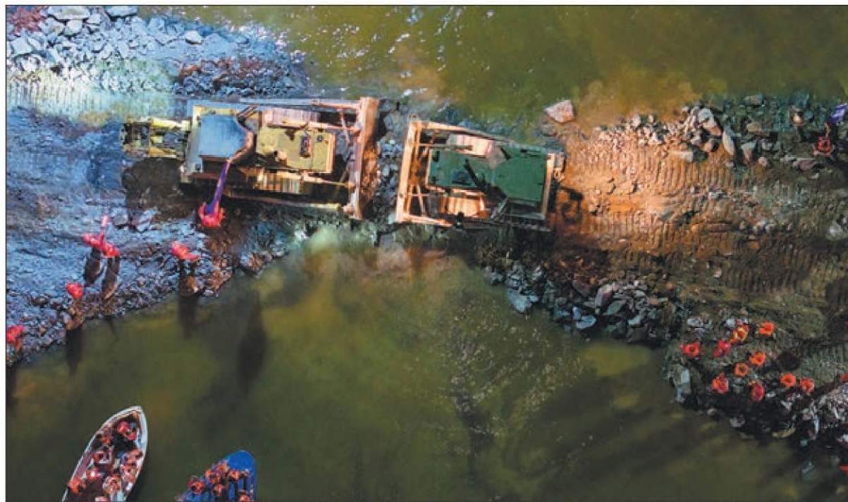
Above left: Rescuers work to block the dike breach next to Dongting Lake in Huarong county, Hunan province, on Monday. As of Monday afternoon, 180.5 meters of the 226-m breach in the dike had been sealed, according to the Yueyang flood control and drought relief headquarters. CHEN ZEGUO / XINHUA Top right: Rescuers drain floodwater from an area near Dongting Lake in Huarong county on Tuesday. CHEN SIHAN / XINHUA Above right: Rescuers try to seal the breached dike on Sunday. CAO BOYUAN / FOR CHINA DAILY
