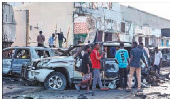
People inspect the damage caused by a car bomb blast outside a cafe on Sunday in Mogadishu, Somalia. Nine people were killed and 20 others wounded when the bomb went off in the place that was packed with soccer fans watching the Euro 2024 final. HASSAN ALI ELMI / AFP
