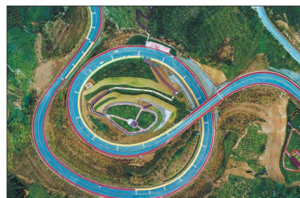
An overhead view of the Yellow River No 1 Highway in Linfen city.
