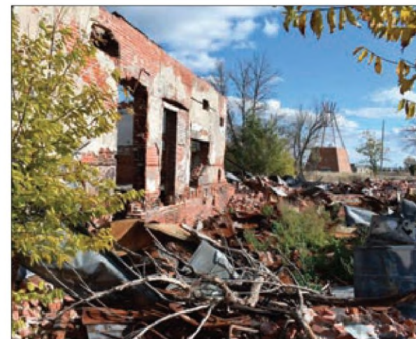
The ruins of a building that was part of a Native American boarding school on the Rosebud Sioux Reservation in Mission, South Dakota, are shown on Oct 15, 2022. Federal officials with the Interior Department called on the US government Tuesday to apologize for a nationwide system of boarding schools in which Native children faced abuse and neglect. MATTHEW BROWN / AP
