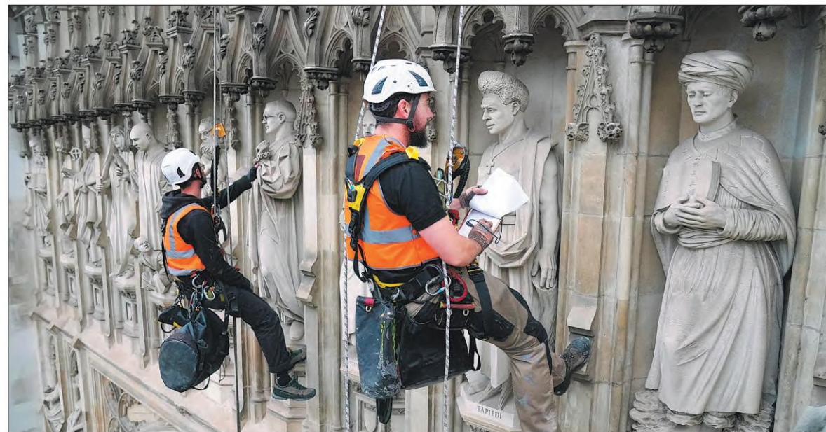
Specialist abseilers conduct an annual inspection of the condition of the stonework of the West Towers at Westminster Abbey in central London on Tuesday. Westminster Abbey, the site of 40 English and British monarchs' coronations, most recently hosted King Charles III's coronation in May last year. PA
