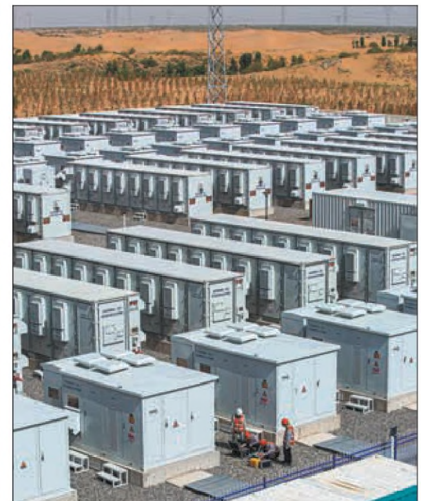
Staff members test the energy storage power station of the Kubuqi 2 million kilowatt photovoltaic desert control project, on June 24.
