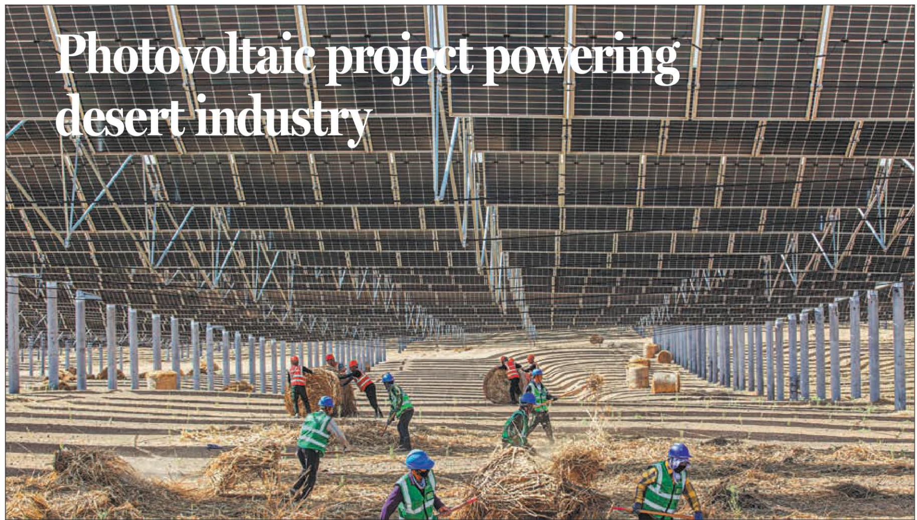
Workers spread dry reed grass under photovoltaic panels to repair and solidify the sand, on June 26. PHOTOS BY MEI TAO / HUBEI DAILY
