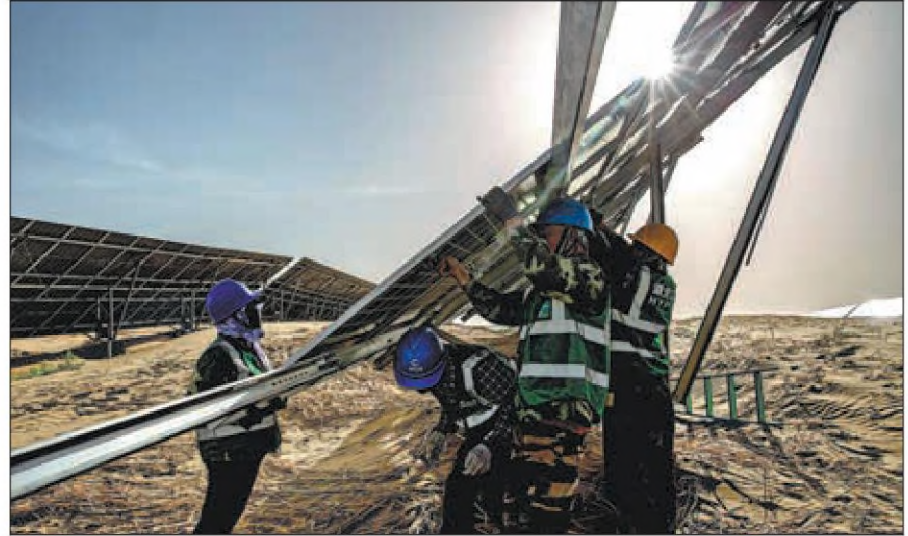
Construction staff members install photovoltaic panels, on June 24.
