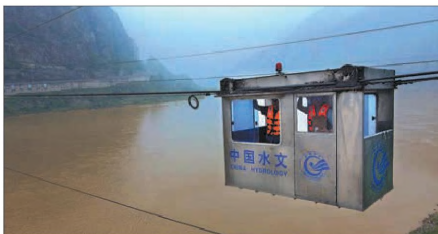
The hanging crane box on the cable path across the Yellow River is the only way to access the station.
