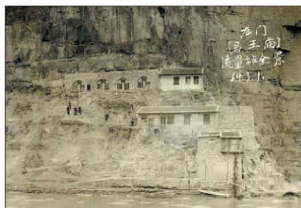
A photograph of the original Longmen Hydrological Station, taken in 1964. PROVIDED TO CHINA DAILY
