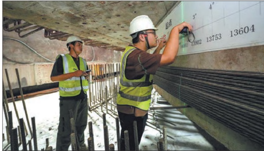
CREC4 builders conduct check on equipment before swinging the world's heaviest asymmetric curved cable-stayed bridge in Jiujiang, Jiangxi province. SHEN JIAPENG / FOR CHINA DAILY
