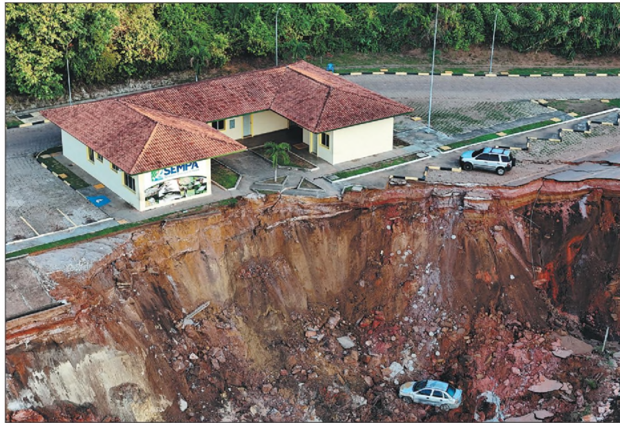
Buildings stand precariously on the edge of a massive crater created by a landslide in Manacapuru, Brazil's Amazonas State, on Tuesday. Authorities estimate about 200 people could be buried beneath the rubble. The cause of the landslide remains unclear, but officials warn that the severe drought in the Amazon region might destabilize riverbanks, leading to further natural disasters. BRUNO KELLY / REUTERS
