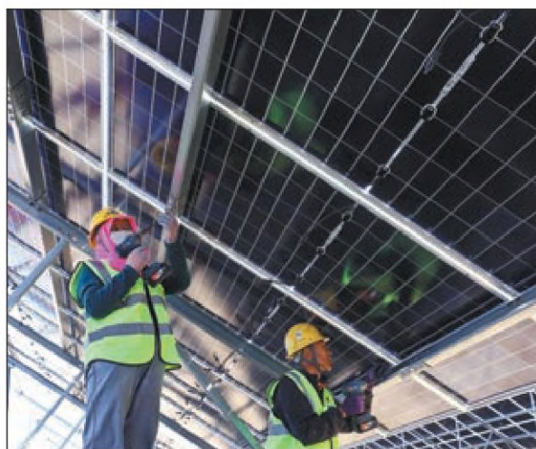
Employees install PV panels at a power plant in Zhangye, Gansu province, on Oct 1. WANG JIANG / FOR CHINA DAILY
