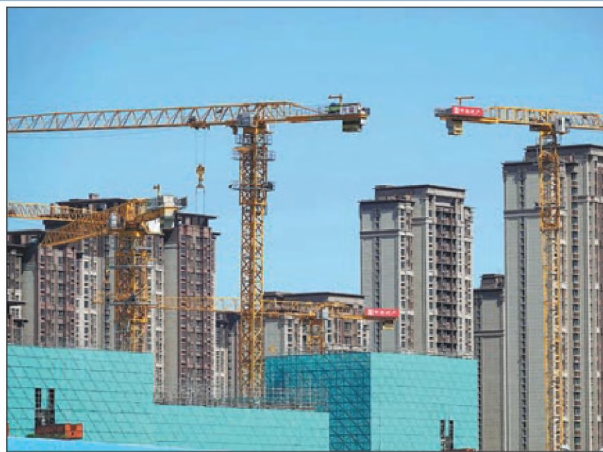
A property project under construction in Beijing. TANG KE / FOR CHINA DAILY
