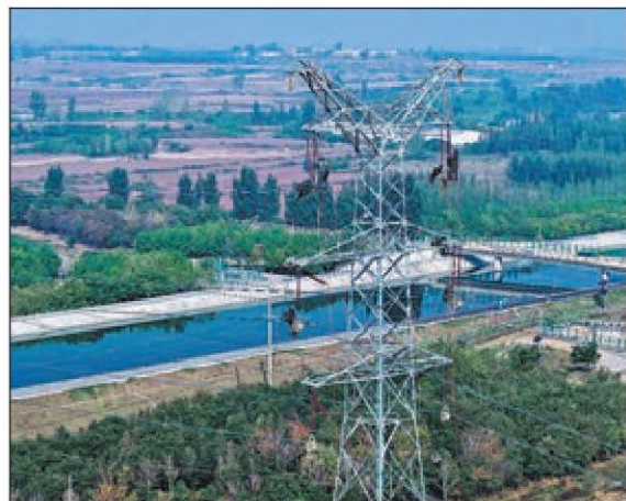
Employees from Henan Anyang Power Supply Co install power line accessories on Towers 5, 6 and 7 of the Wenfeng-to-Juyuan 220 kV line project on Wednesday in Anyang, Henan province, aiming to boost power supply in the city's northwestern areas. ZHANG YANG / FOR CHINA DAILY
