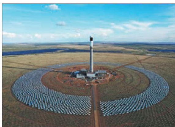
A view of a Chinese-invested power project in South Africa.
