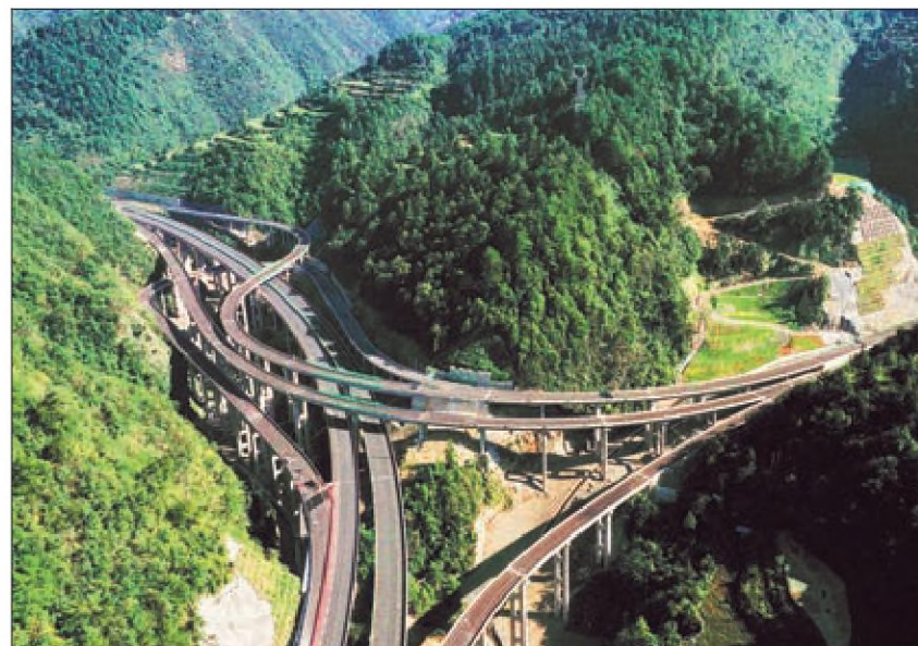
A photograph taken by a drone shows an aerial view of the Jianhe-Liping expressway in Guizhou province last week. Construction of the vital local passageway in the mountainous province was undertaken by major State contractors such as China Railway Construction Corp's 17th, 18th and 24th bureaus. The north-south expressway opened to traffic on Friday, shortening travel time between Jianhe and Liping counties from three hours to about one hour. PROVIDED TO CHINA DAILY
