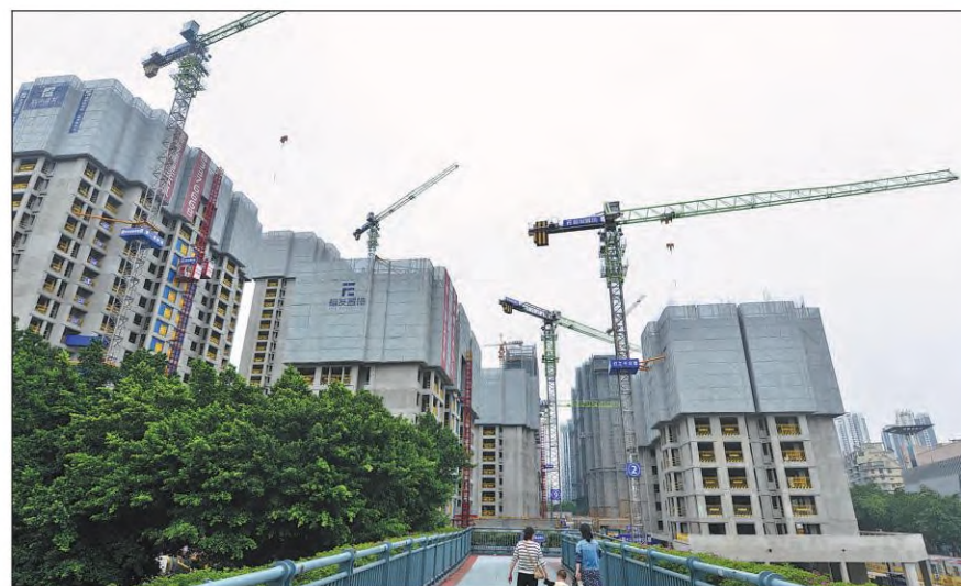
A residential project under construction in Fuzhou, Fujian province, on April 16.
