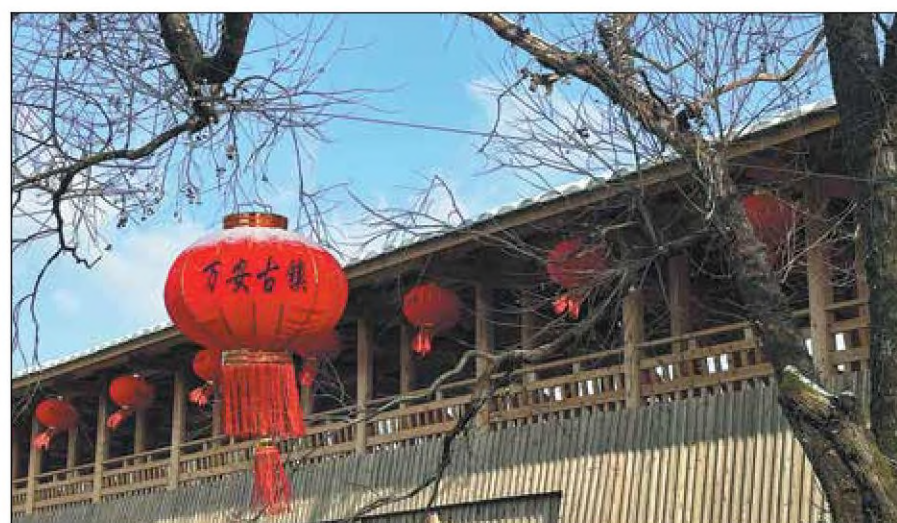
After severe fire damage in 2022, Wan'an Bridge displays its extensive restoration by the Huang family last year. PHOTOS PROVIDED TO CHINA DAILY
