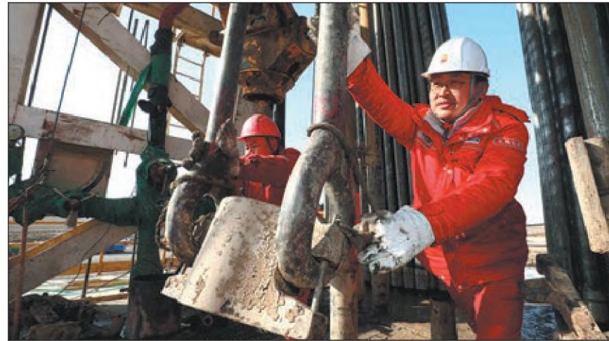
Employees work at PetroChina GWDC's No 2 Drilling Co's construction site in Shuang 229 block of Liaohe Oilfield in Liaoning province. By integrating green development into the whole process of oil and gas exploration, they have drilled 108,049 meters of wells so far this year, with zero pollution to the environment. LIU CHUANBAO / FOR CHINA DAILY
