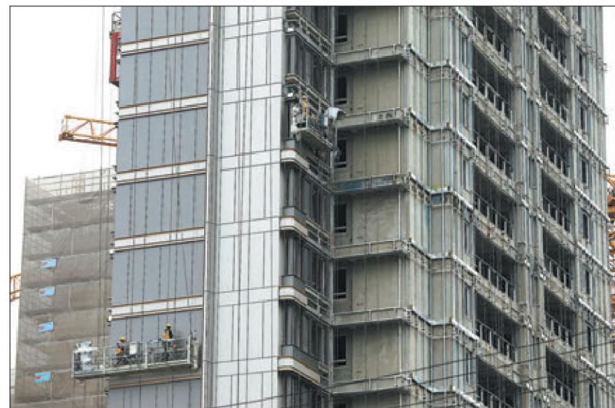
A building under construction in Shanghai. PROVIDED TO CHINA DAILY
