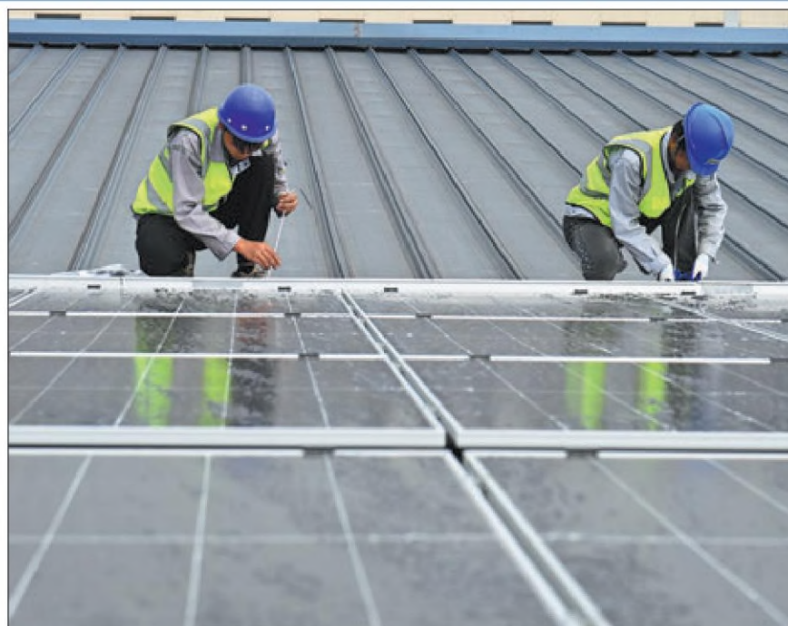
Technicians install photovoltaic panels in Chongqing. SUN KAIFANG / FOR CHINA DAILY
