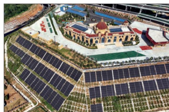
Photovoltaic panels are installed along the Jiwei (Jinan-Weifang) Expressway in Shandong province. PHOTOS PROVIDED TO CHINA DAILY
