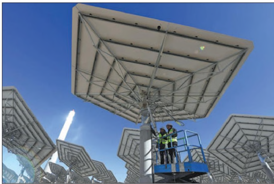
Technicians check equipment at a solar power station in the Kazak autonomous county of Aksay, Gansu province, in November. TIAN YUE / FOR CHINA DAILY
