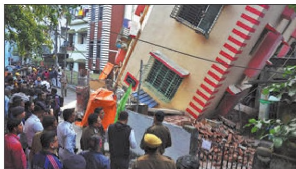
A four-story building tilted precariously in Vidyasagar Colony, Baghajatin, Kolkata, India, on Tuesday. Preliminary investigations revealed that inferior quality materials were used in the construction of the building. DEBAJYOTI CHAKRABORTY / GETTY IMAGES
