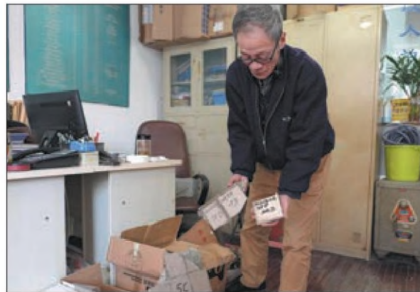
Left: Maintenance worker Liu Shouliang displays tiles that had fallen off the Zhaofeng Building over the years. Right: Bao Lei (left), Party chief of the residential community where the building is located, and resident Liu Guanglei (right) share their insights on how the self-funded renovation project came into being.
