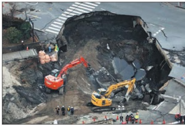
Rescuers work at the site of a road collapse on Sunday in Yashio city, Saitama Prefecture, near Tokyo, where a growing sinkhole swallowed a 74-year-old truck driver. Authorities suspect corroded sewer pipes caused the collapse. THE YOMIURI SHIMBUN VIA AP
